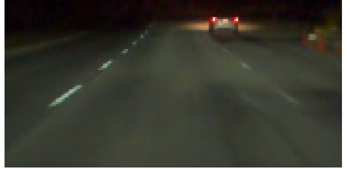
Fig. 6: A frame that caused the conformance test to fail due to the faded right-hand lane line
